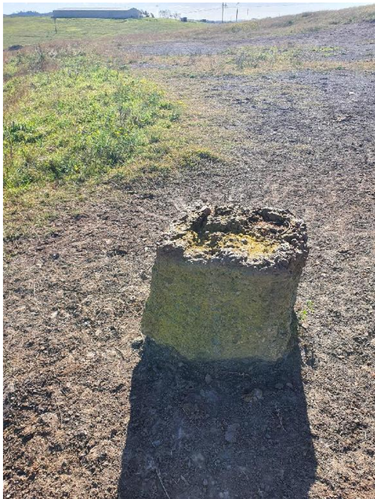
Photo 123 - Footing, Former Structure (MRP109)
