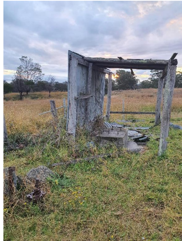
Photo 26 - Structure (Possible Pump House) (MRP23)
