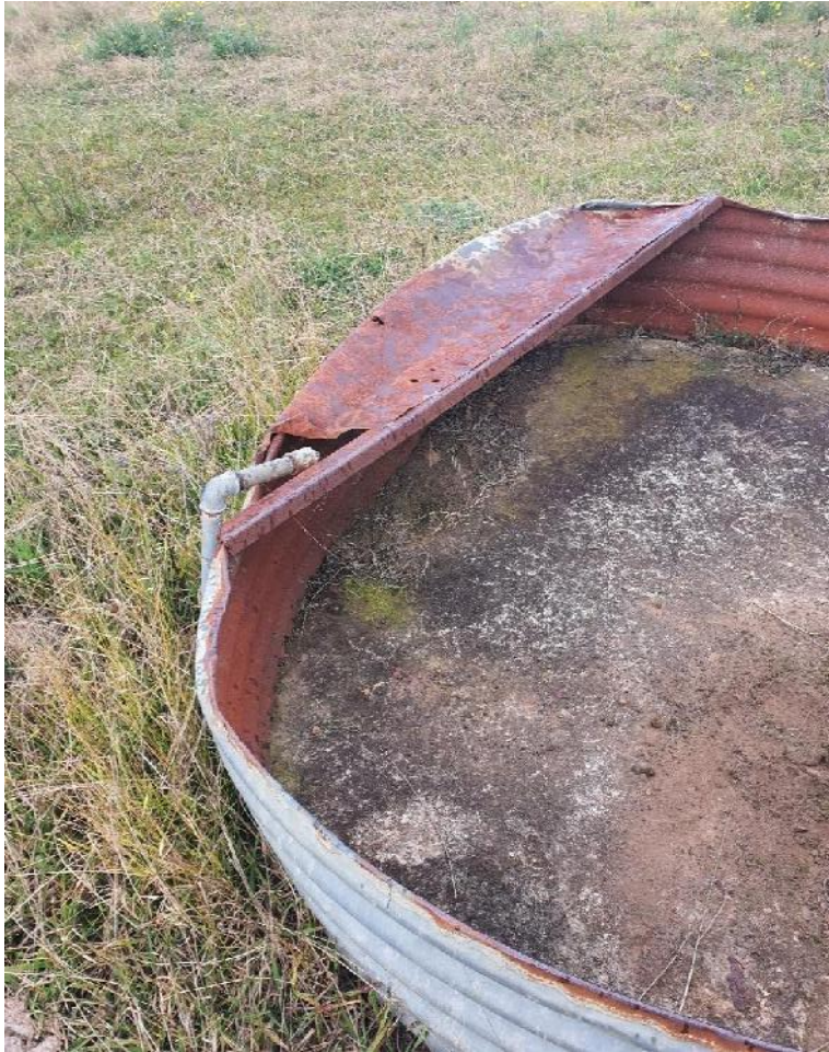
Photo 7 - Trough with Steel Pipe Inlet Riser (MRP7)
