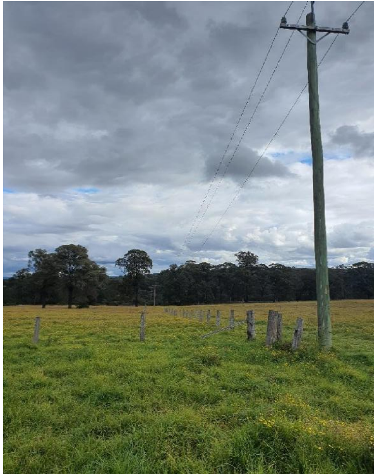
Photo 15 - Power Poles (MRP13)
