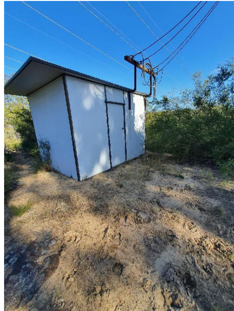
Photo 134 - Shed and Coalwash Road (MRP117)
