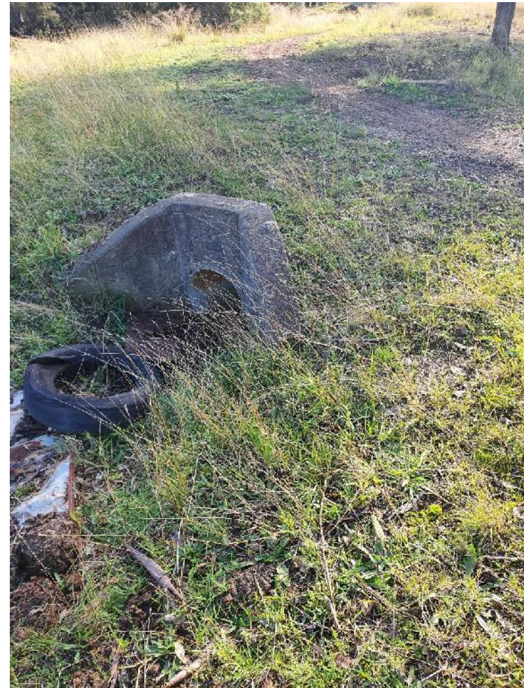
Photo 66 - Concrete Headwalls and Pipes Along Road (MRP58)
