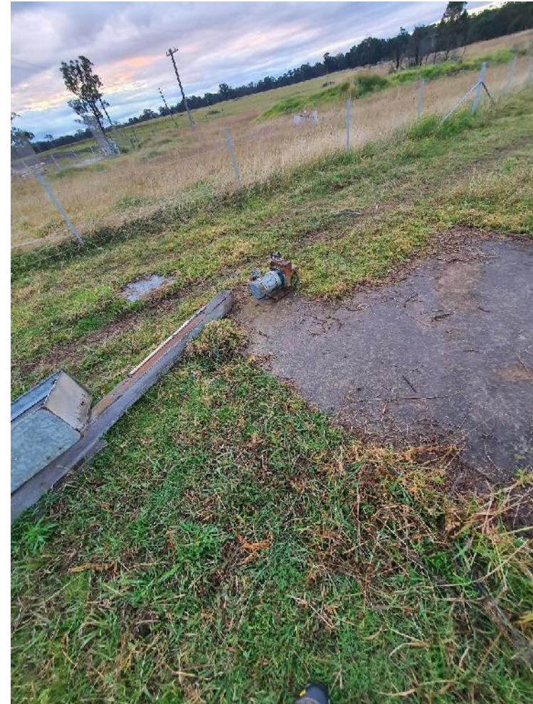
Photo 22 - Slab Pump and Meter Box (MRP18)
