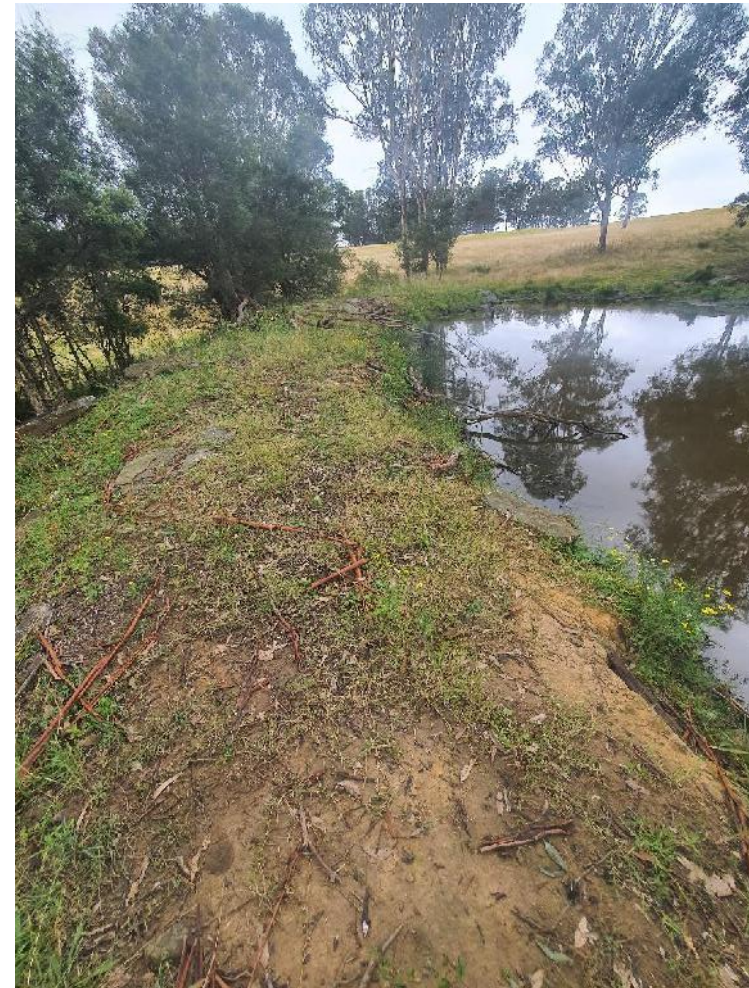
Photo 44 - Dam Embankment (MRP37)
