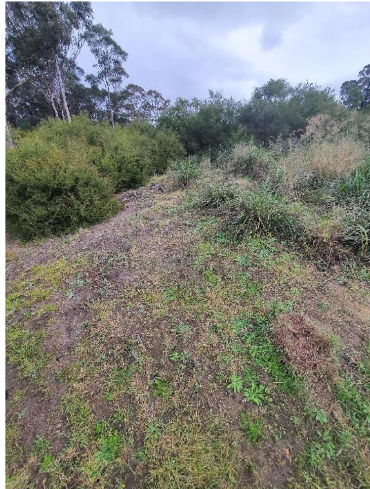
Photo 54 - Filled Ground (MRP47)
