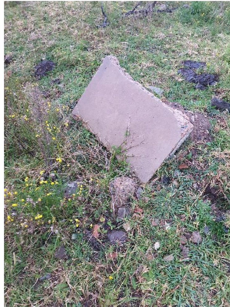
Photo 28 - Building Rubble (MRP24)
