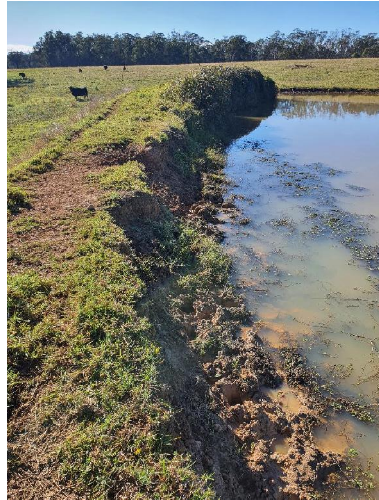
Photo 30 - Dam Wall (MRP25)
