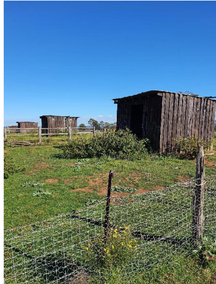
Photo 36 - Timber Structures (MRP32)
